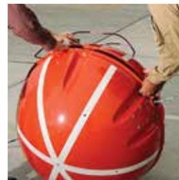
This makes it possible to install markers on otherwise inaccessible lines across rivers or deep canyons, or where it is not feasible to take the line out of service.
